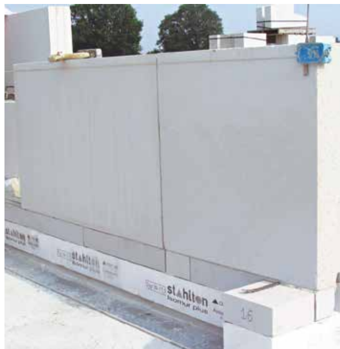
Elements laid as the bottom layer in brickwork
