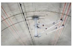
This is executed with high precision, as is the case with anchor channels used for concrete tunnel linings. These channels are checked with gauges specifically for your site.
