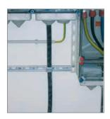
Cold-formed JORDAHL® mounting channels can be used for a multitude of static loading conditions, e.g., to fasten pipes, cables, etc.
