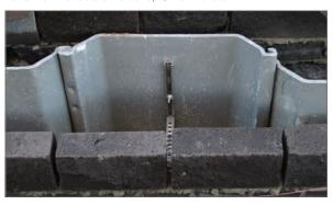
Connection of brickwork to sheet-pile wall.
