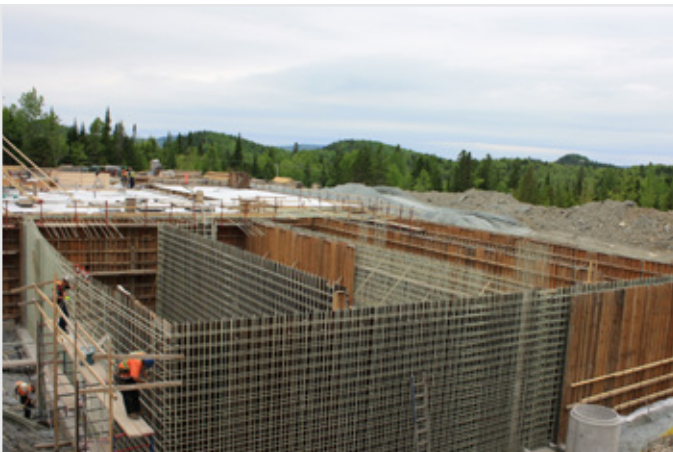
Tanks for sewerage treatment plant, slab- and wall reinforcement
