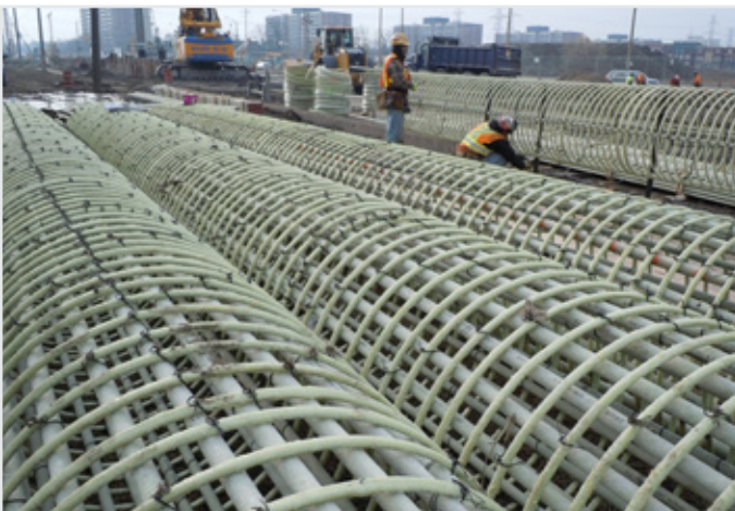
Reinforcement cages made of straight and spiral-shaped FIBERNOX® V-ROD reinforcement
