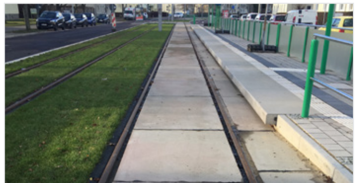
Steel free tramway cover slabs, Magdeburg, Germany
